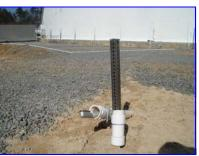
Bore pits and trench excavations are back-filled and site is cleaned.
